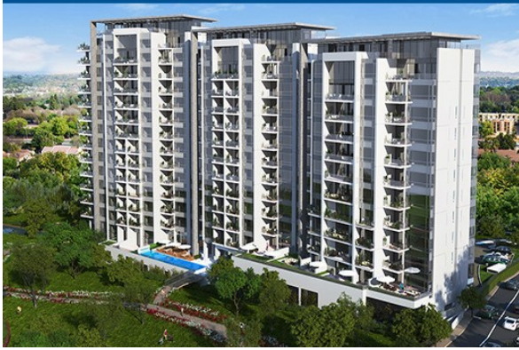
Metropolis on Park - Sandton
